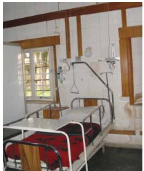
Intensive Care Unit of K-1 Hospital.
