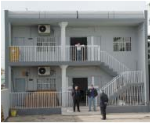
Looking over the new clinic building
